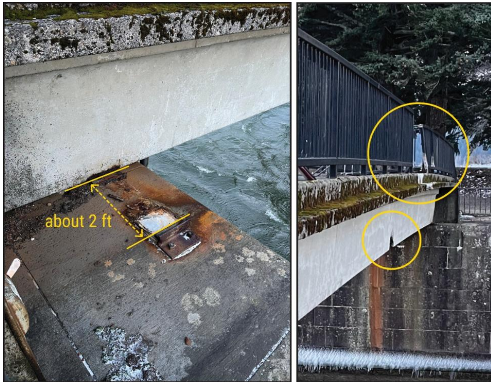
Figure 6. Left to right: Markings showing the displacement of the deck of the Thunder Island pedestrian bridge, and further damage to the deck and railing (circled). (Background source: Port of Cascade Locks Port Commission)
