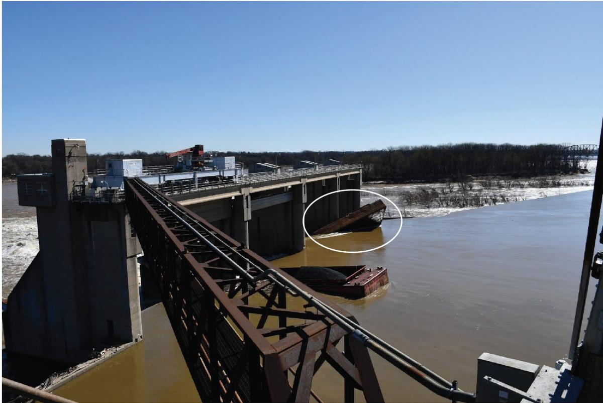
**Figure 5.** Barges from the *Amber Brittany* tow lodged in the Lower McAlpine Dam Gate after the tow broke apart.
